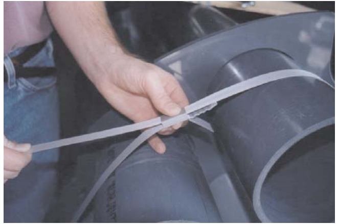
8. Place a seal over both ends of the strap. The seal should not interfere with the folded over end of the strap.
