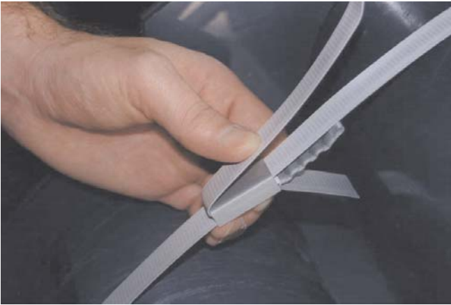
9. Take the slack out of the strapping, then fold the upper strap end back as shown. This fold will normally keep the strapping snug while performing step 10.
