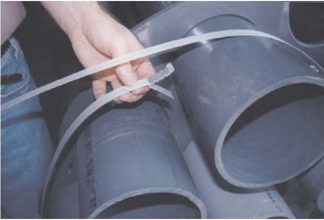
7. Pull the strap with the pre-assembled seal around conduits as shown.
