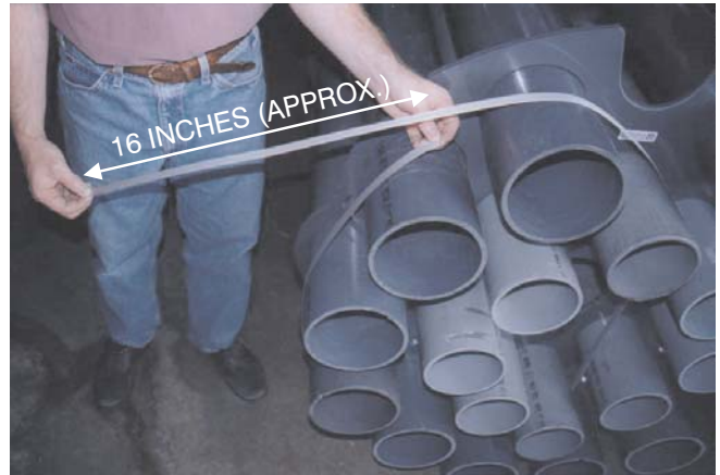
2. Cut off a length of strapping that is approximately 16 inches longer than the distance around the conduits being secured.
